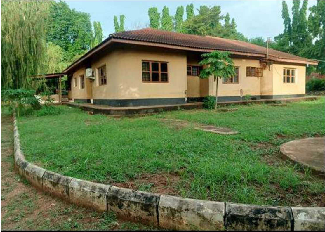
Plate 2.2: The Main building (OUT Regional Centre Office)
