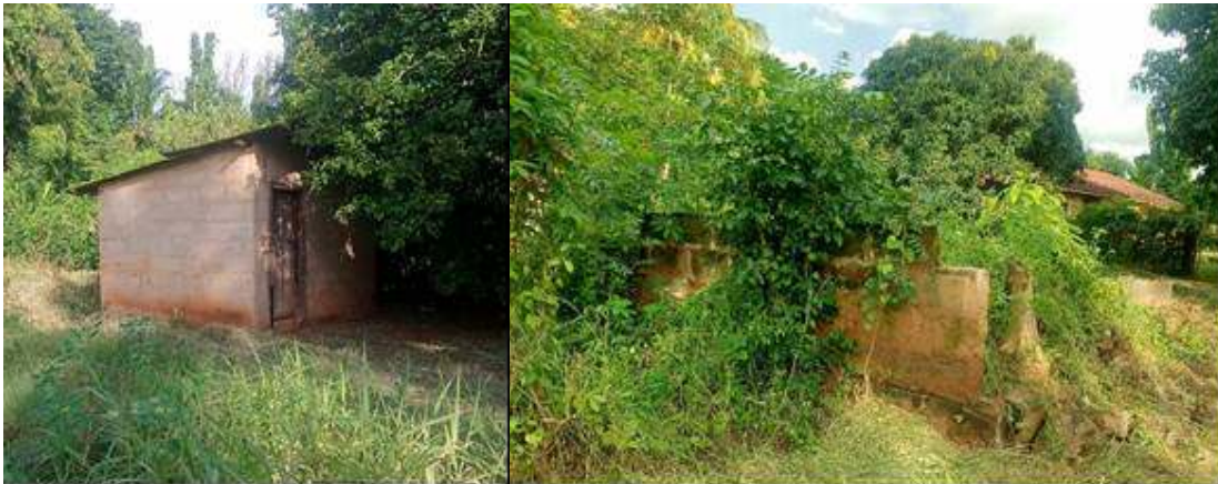
Plate 2.3: Existing structures in site
